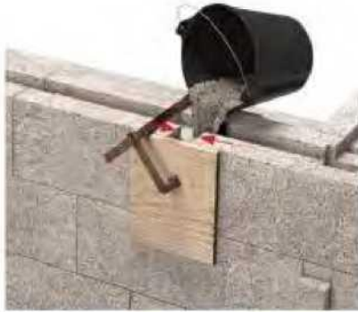
Figure 30: assembly of running wall with space less than 10 cm (4 in.) remaining
