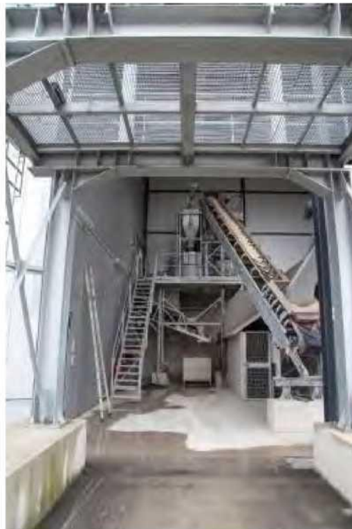
Figure 19: concrete block center
